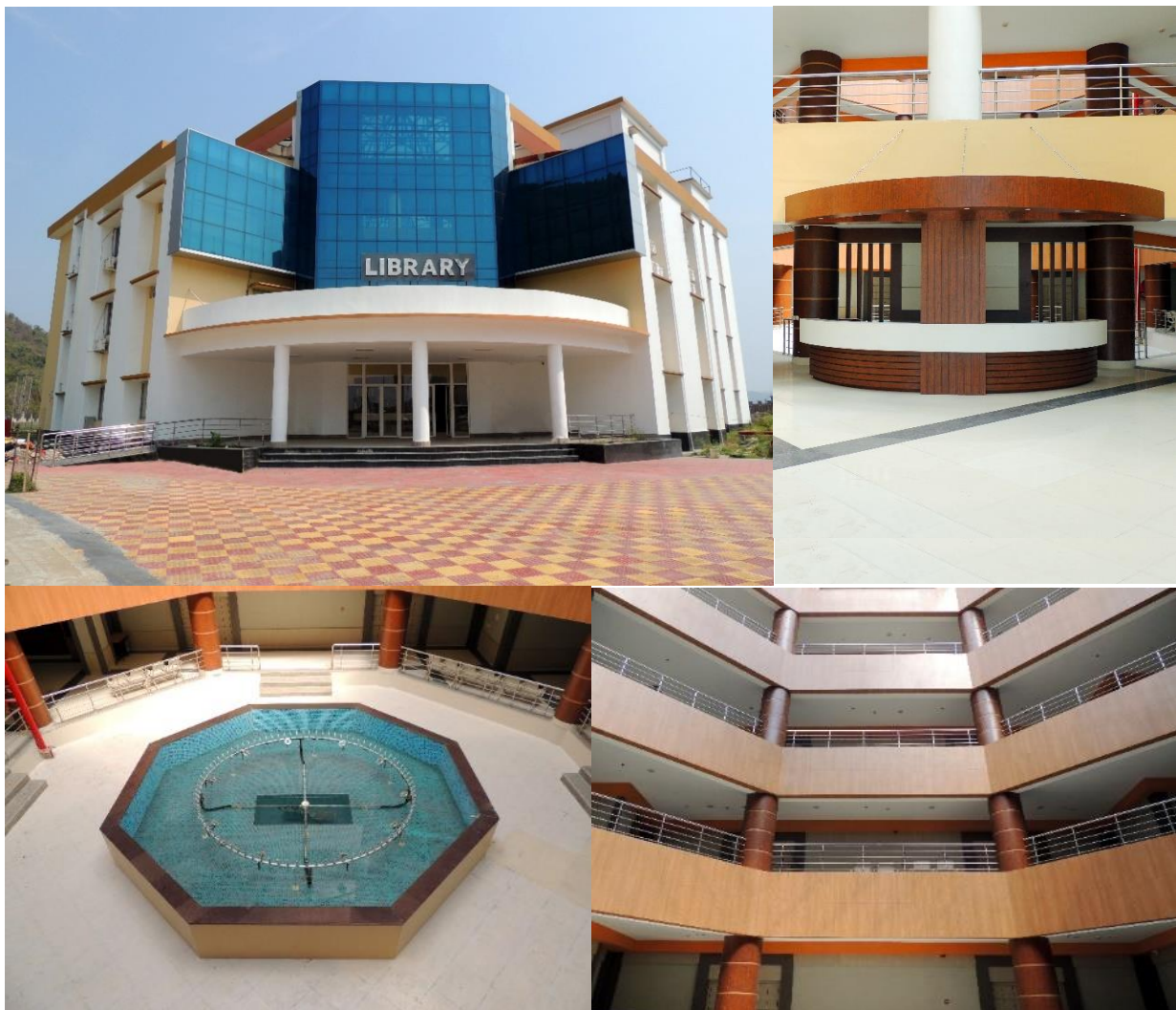
Pictorial collage of newly constructed Library
